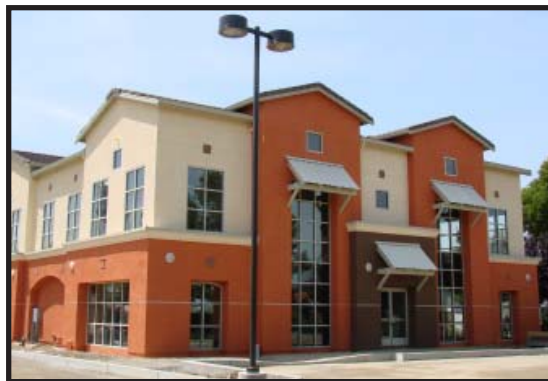
Newly constructed West Park Executive Suites
